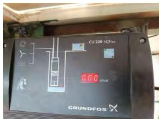
Figura 76 – Panel de control de bombeo – Pellel.
